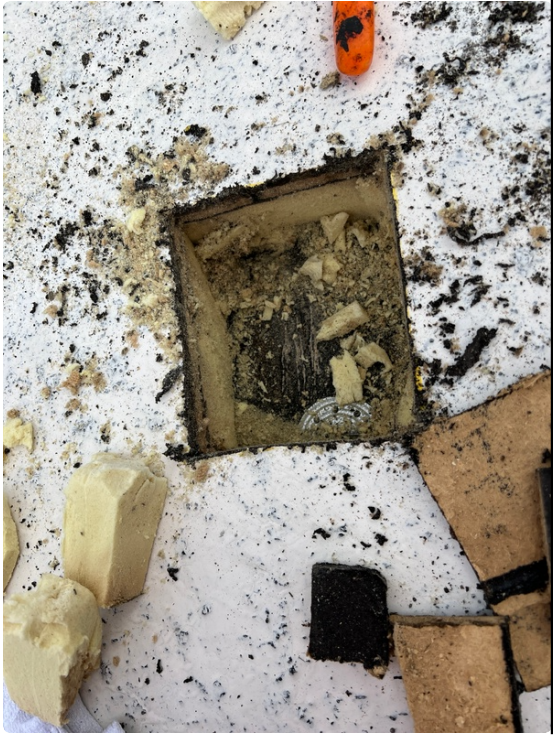
View of core cut hole. SBS nailable base sheet can be observed
