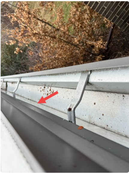
New gutter bracket to be fastened 2" higher then bottom of edge metal and sealed with sealant.
